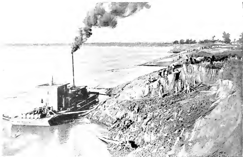
SLOPING THE UPPER BANK WITH HYDRAULIC GRADER.
